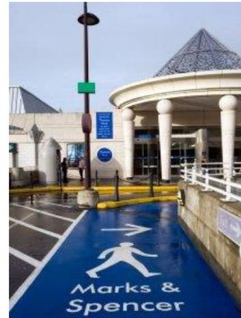
Way-Finding is a simple way to help car park users locate shops, pay stations and their car. Way-Finding can be in the form of a colour coded pedestrian walkways which have directional arrows and text to guide the user to a particular destination. Virtually any colour and font can be created for Way-Finding and anti-slip properties can be added to paints to ensure walkways are non-slip.
